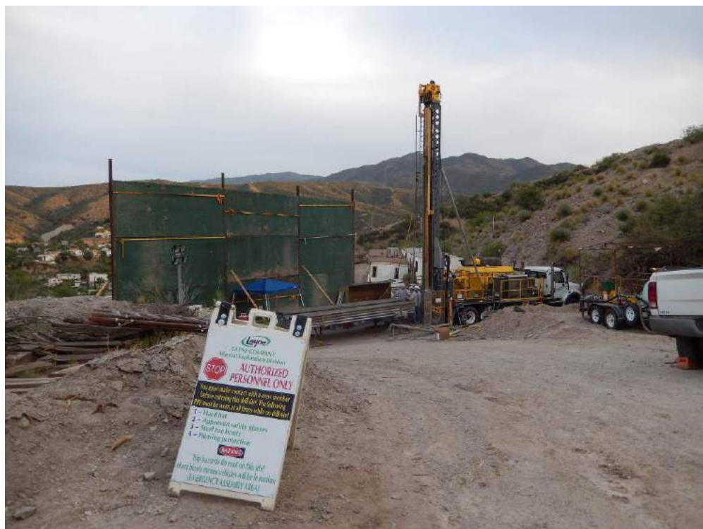
Plate 10-1 Large Sound Barrier Erected to Reduce Impact of Drilling for Local Residents, Hole VD14-01
