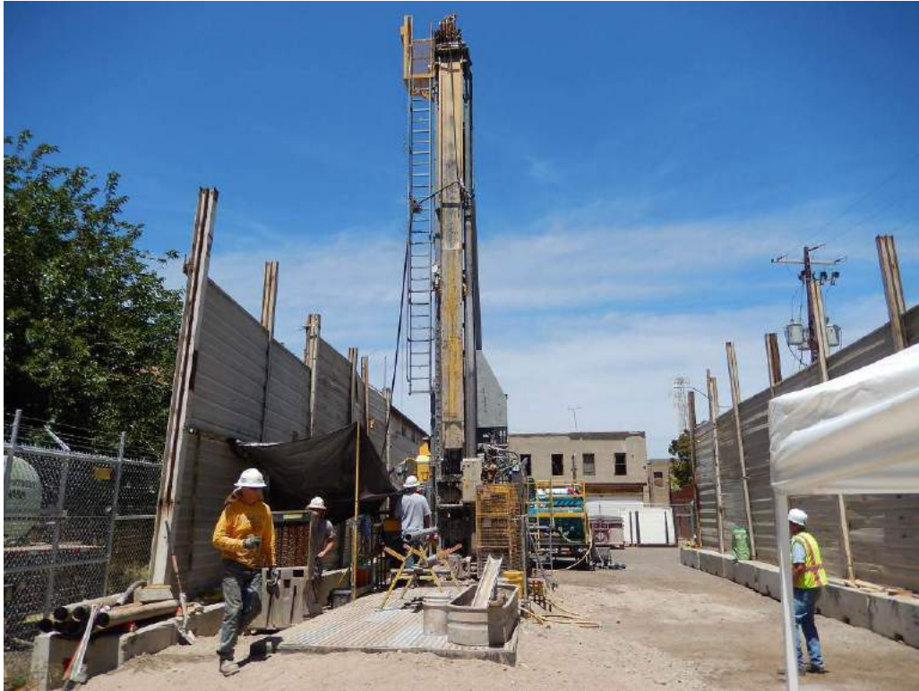
Plate 10-2 Drilling of Hole VD14-06 from a Parking Lot Located in the Center of Miami, Arizona
